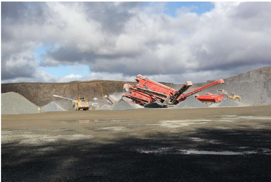
Figure 3.3 – Secondary processing plant
