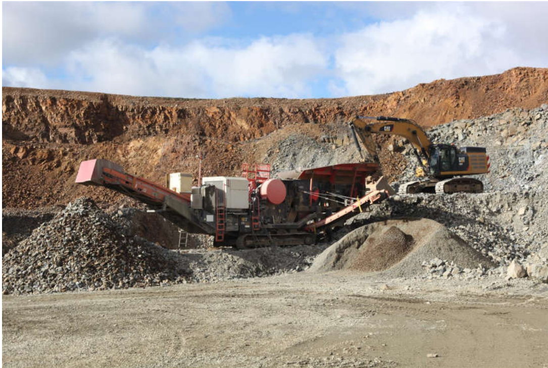
Figure 3.2 – Primary processing plant
